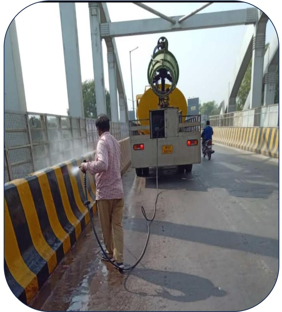
Cleaning of Footpath and Commercial area Through Water Jetting Machine
